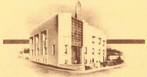
OFFICE: AMADOR COUNTY AIRPORT BLDG. SUTTER HILL
